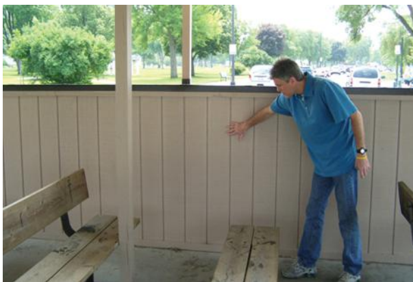
Figure 13.14 On June 8, 2007, after comparing the wall with photos taken in October 2006, Gannon indicated the precise spot on the wall where the significant graffiti had been just days before. The smell of fresh paint was in the air.
