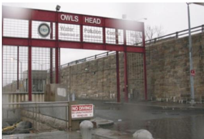
Figure 3.6 The area in which Larry Andrews was recovered on February 12, 1998, was just to the left of the entry gate to Owls Head Water Pollution Control Plant. This was the same location where Pat McNeil had been recovered almost a year earlier on April 7, 1997.
