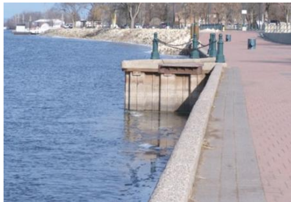
Figure 15.9 The levee in La Crosse presented an abrupt drop off of 6 feet. Luke Homan was recovered near where this photo was taken and about 20 feet out from the levee.
